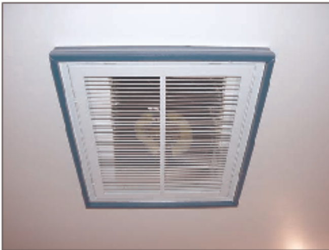
Figure 4.6a — Silent duct boot, grille closed
